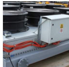
Electric connection box.
