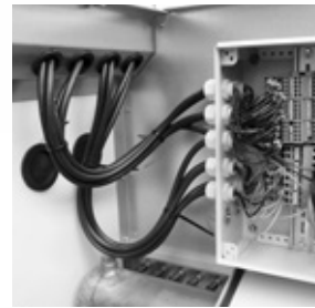
Common terminal box for motors.
