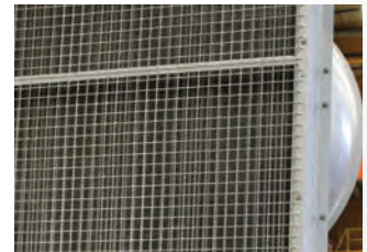
Fin surface protection grid, mounted on cooler air intake side.
