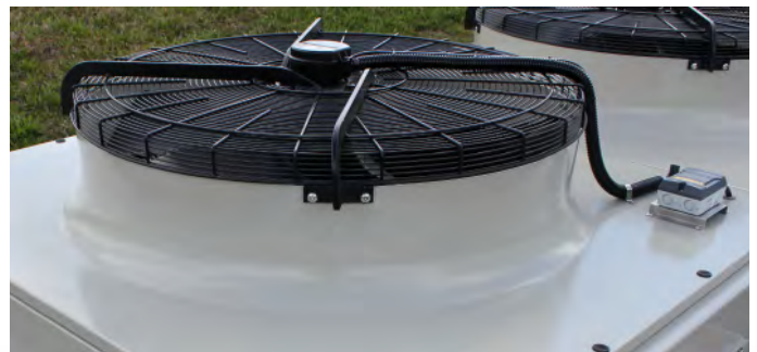
The coolers could be ordered with external- or internal rotor motor technology.
