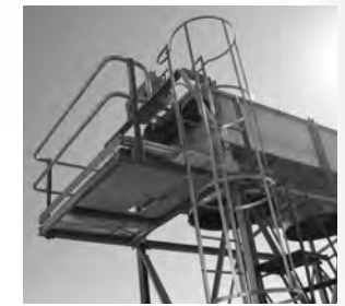
Railing, ladder & maintenance platform.
