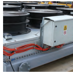
Electric connection box.
