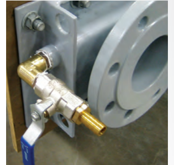
Drain valve QLKZ-04-21.
