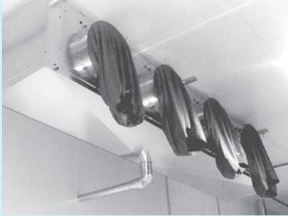
The “Shut Up®” system is used in industrial cubic unit coolers: it consists of special open textiles ducts that are fastened to air outlet fan shrouds. These “socks”, by their nature, sag when the fans are turned off, folding down on the motor and creating a thermal barrier that significantly reduces both the duration of the defrost cycle and temperature fluctuations in the cold room.
