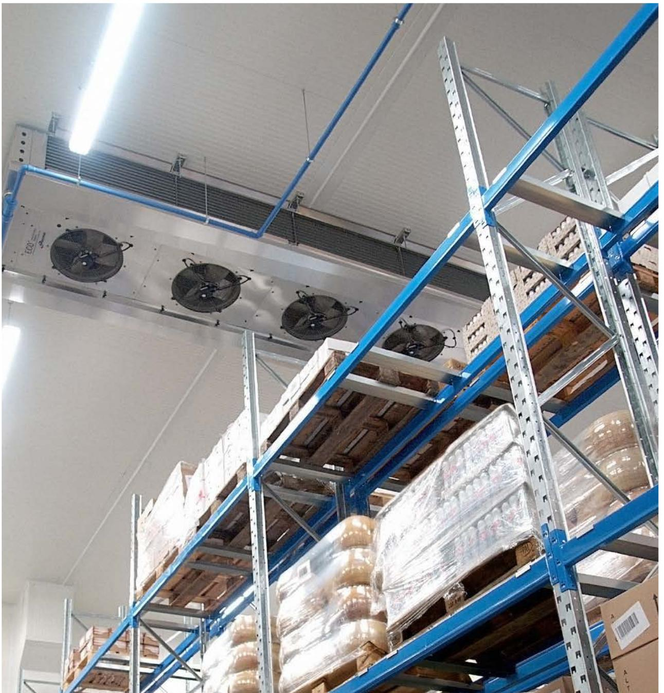
Unit coolers / Air cooled condensers / Dry coolers
